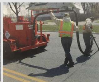
Crack Seal
