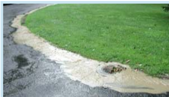
Sediment being carried to storm drain. This could be discharged directly to a stream
