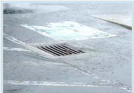
Storm water runoff in a paved parking lot.
