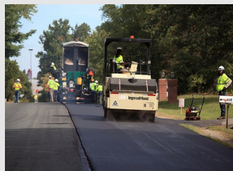
Asphalt Overlay
